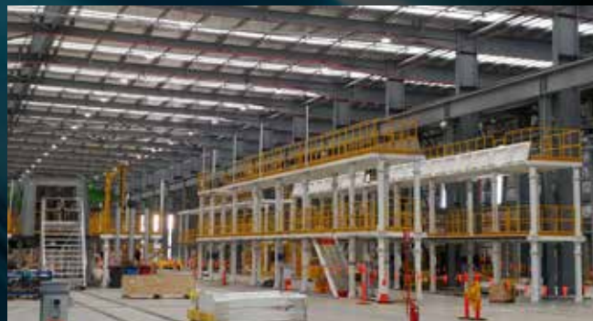
The fitting line being set up at the Bellevue facility.
